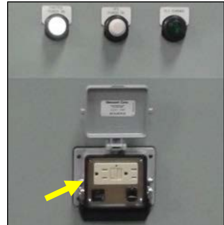
Figure 3-8. Panel Interface Connector
