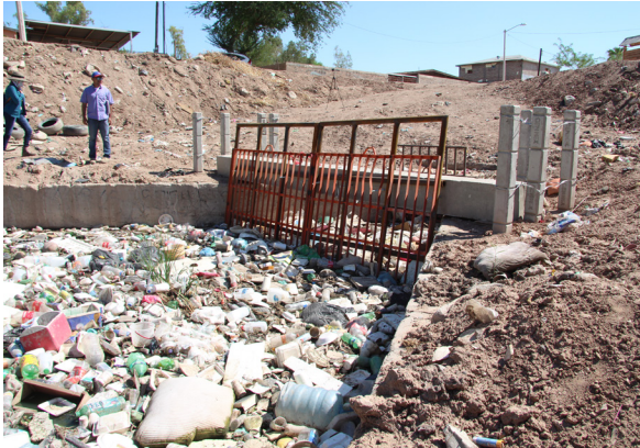
Trash trap at International Drain.
