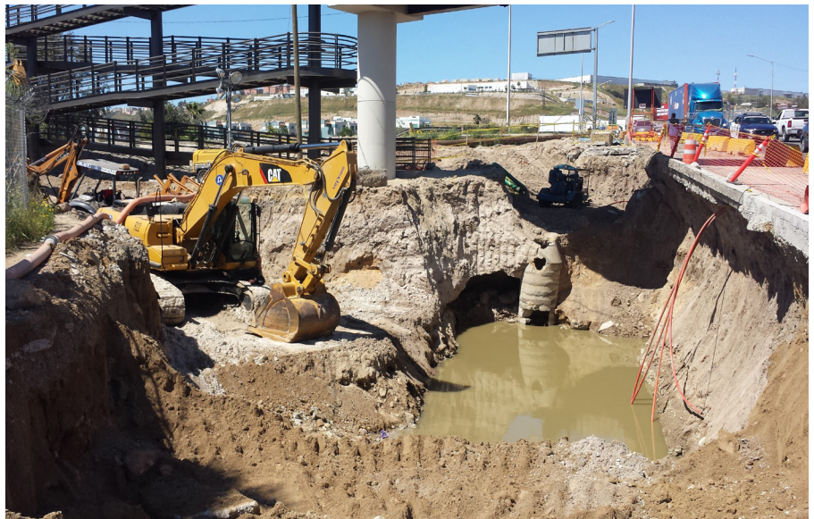
Sewer collection pipe in repair, after collapse. Tijuana, MX. March 29, 2017.
