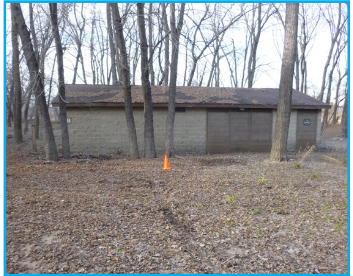
One of the on-site bath houses.
