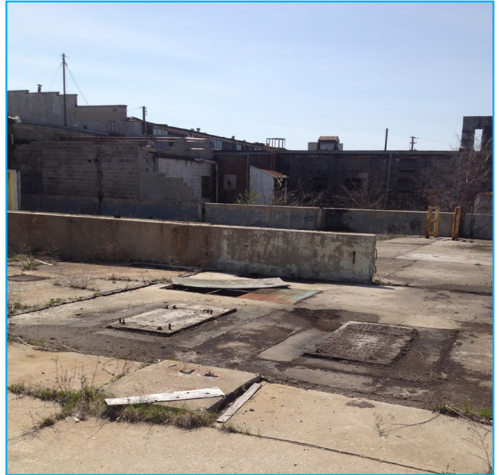
Former SK Hand Tool facility.
