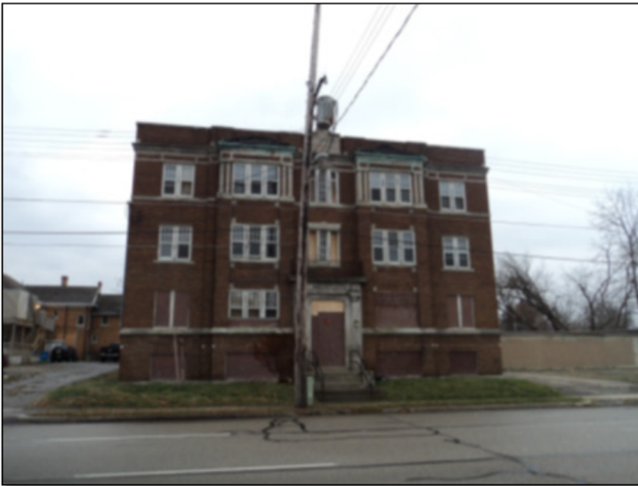
Pre-rehabbed Swayze Apartment building.
