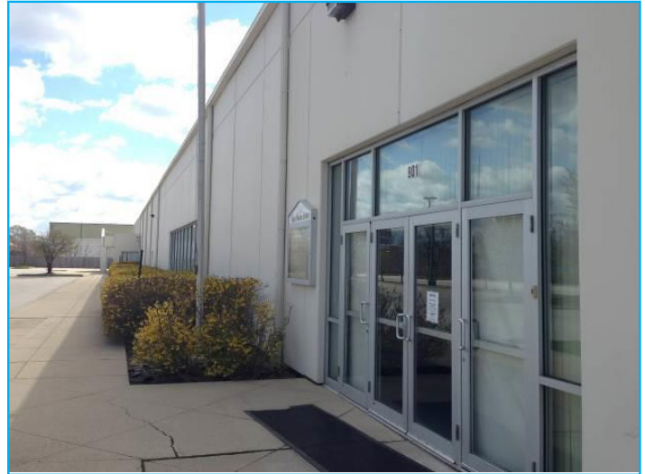
Exterior of a building located on the property.
