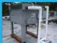
Air-Cooled Heat Exchangers
