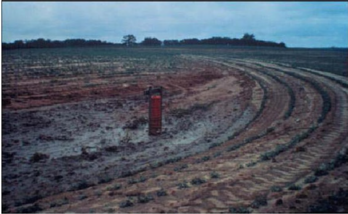
Figure 18. Water and sediment control basin (USDA Natural Resources Conservation Service).
