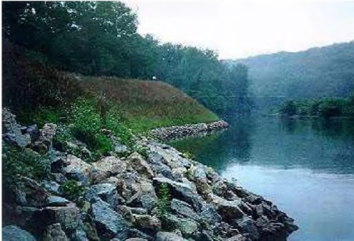
Figure 15. Riprap bank armoring for channel stabilization, Little Miami River, Ohio.
