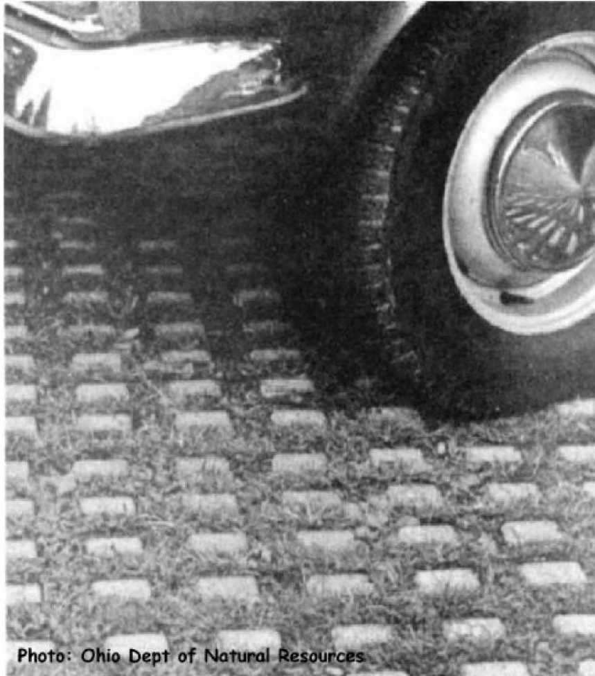
Figure 5. Example of a concrete grid pavement used in an overflow parking area (ODNR 1992).
