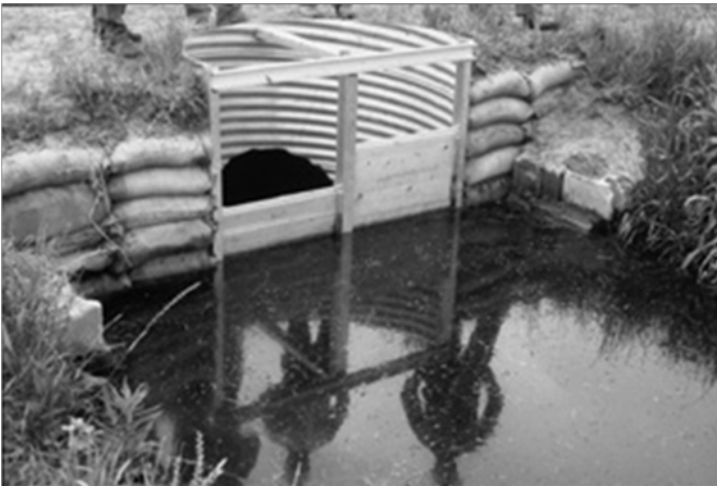
Figure 7. Flashboard riser (Source: http://www.soil.ncsu.edu/publications/BMPs/drainage.html )
