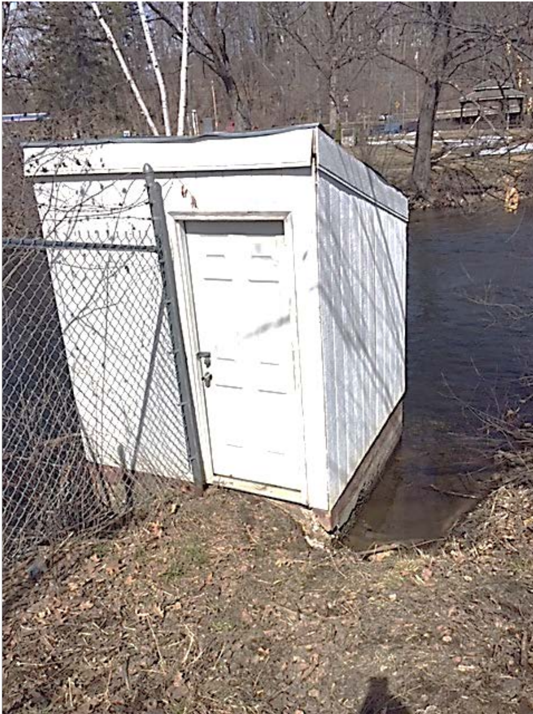
Figure 6: Wooden Shed Covering Cooling Water Intake Structure Sump
