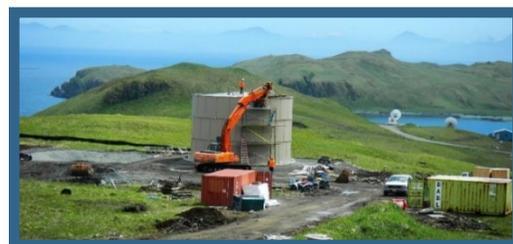
Construction of the 163,000-gallon water storage/disinfectant contact tank in Atka, AK
