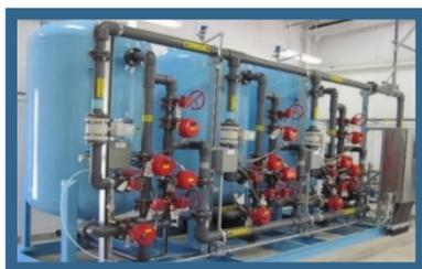
Greensand filtration water treatment plant for the removal of iron, manganese, and arsenic.
