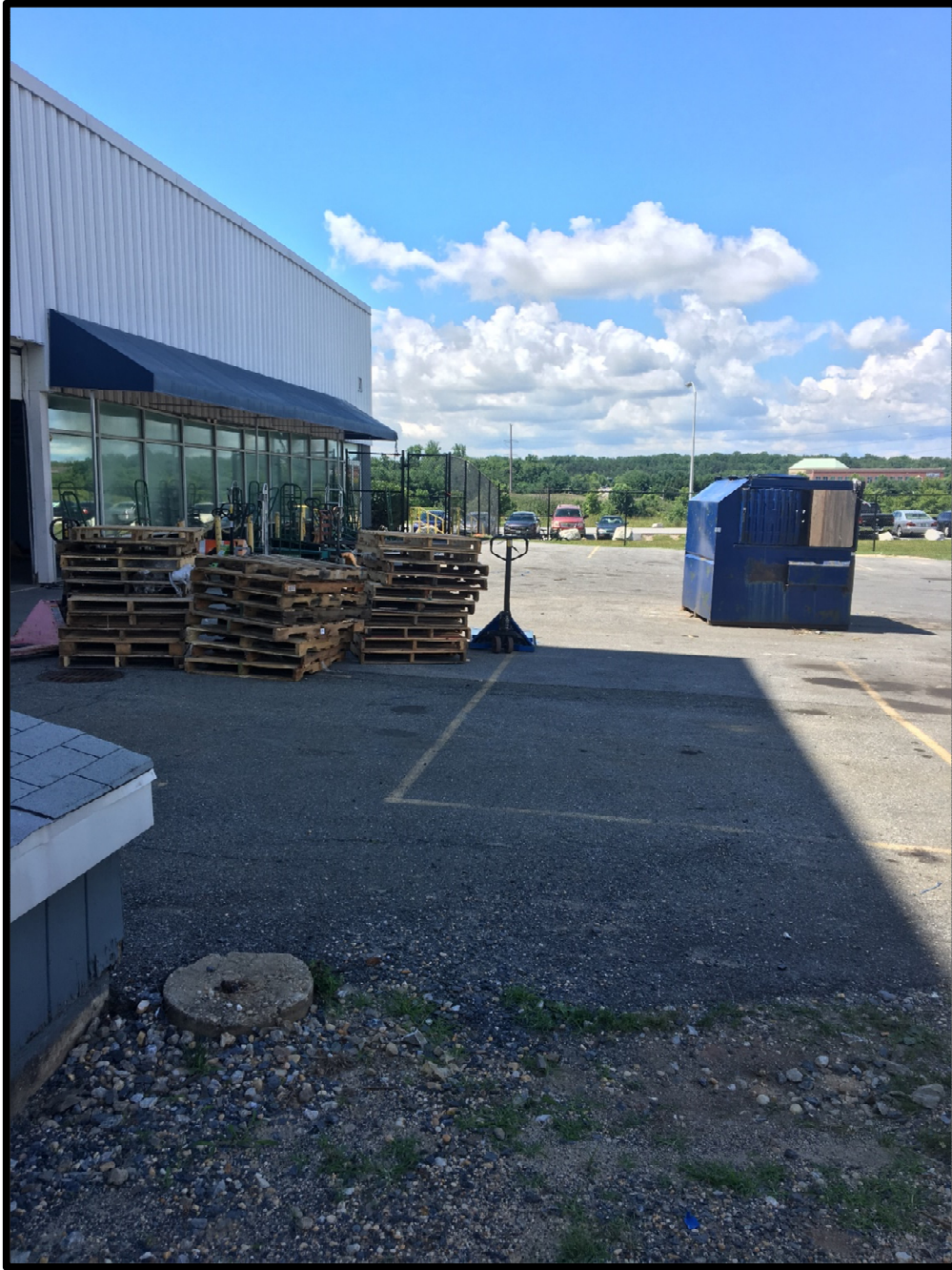
Picture 6: Unit 2 - Former Exterior Trichloroethene Tank Area
