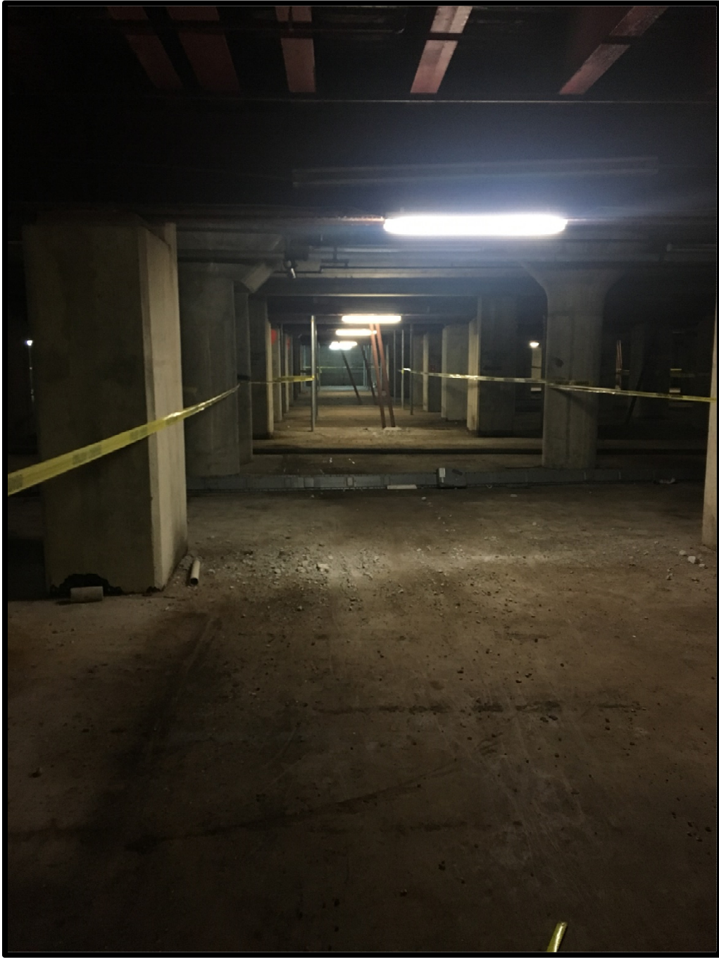
Picture 7: Unit 7 - Press Pit
