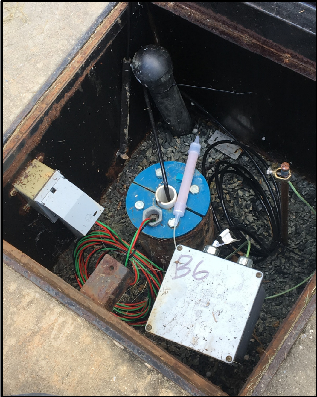
Picture 5: Extraction Well B6
