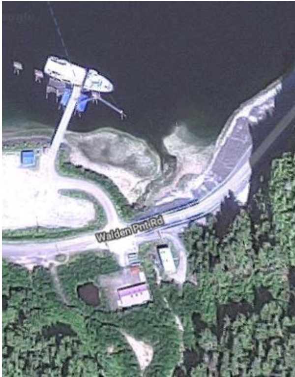
Figure A1: Aerial photo of the Metlaktla Water Treatment Plant
