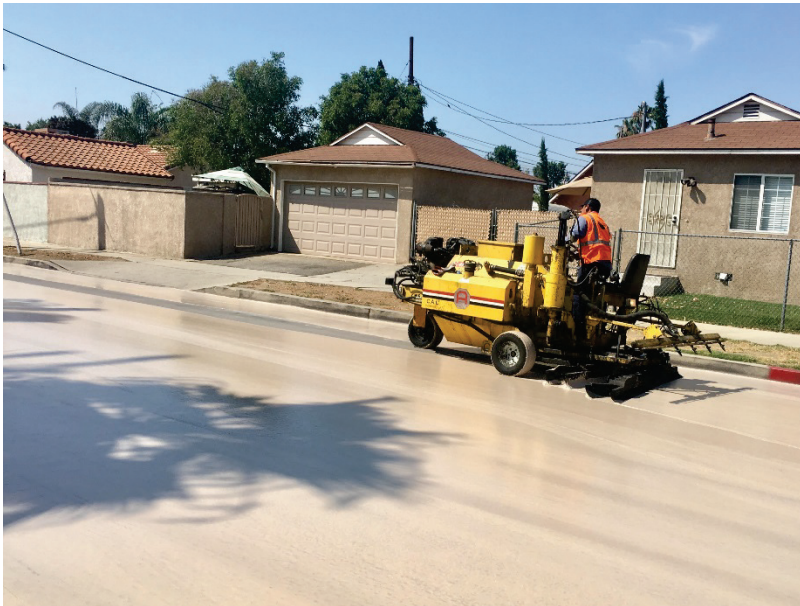
First coat applied using slurry buggy
