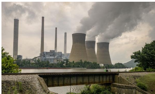
Power plant in Poca, West Virginia. (EPA photo)
