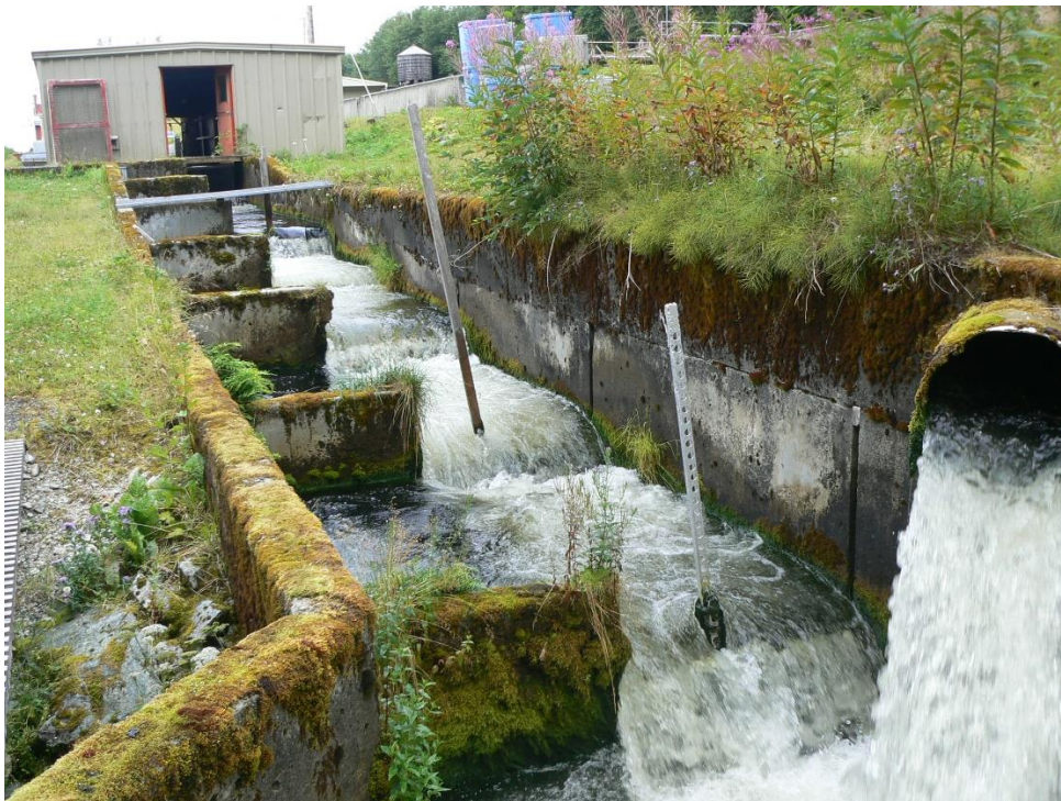
Figure 3: Photograph of Outfall: fish ladder (left) and discharge pipe (right).
