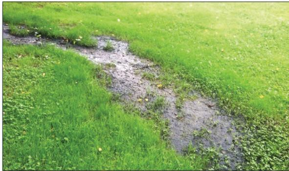
Figure 2. A failing septic system along Hedden Branch.
