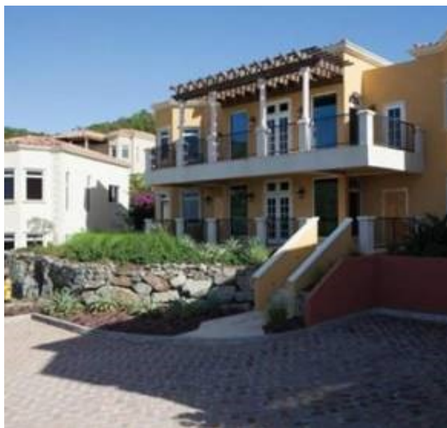
"J" units at Sirenusa, St. John. Unit where pesticide was applied is lower—unit where residents were injured is above.
