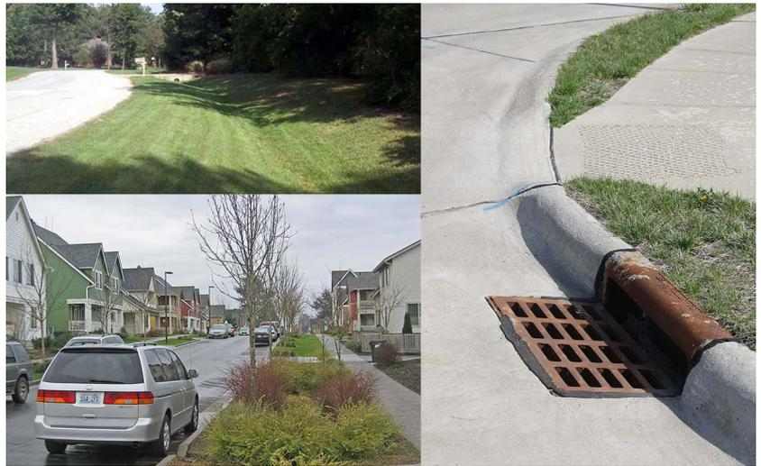
**Green infrastructure, such as vegetated swales (top and bottom left), can reduce costs associated with traditional gray infrastructure, such as a curb and gutter (right)**
