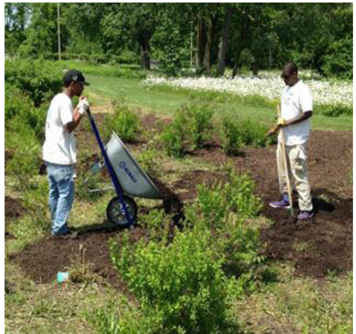
The Onondaga Earth Corps is an established public engagement group that involves local youth in activities such as building and maintaining stormwater infiltration facilities around Syracuse, New York. Barry Tanning, Tetra Tech
