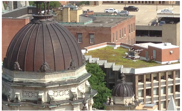
Green roof in the combined sewer area of downtown Syracuse. A wide range of stormwater projects in this area have reduced CSO overflow events and volumes in recent years. Barry Tanning, Tetra Tech
