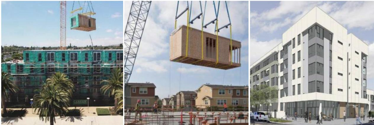
Figure 3. Case study examples of FBH modular residential construction in California.
