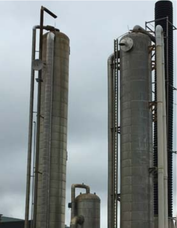
Site visit to Fair Oaks Farms in Fair Oaks, IN, in September, 2018. The anaerobic digesters convert manure into biogas that is then refined into compressed natural gas (CNG) to fuel the milk trucks and to generate electricity to power the farm buildings and machines. Surplus clean biogas is piped and sold to a CNG fueling station.
