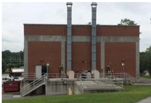
Atlanta's R.M. Clayton Pump Station was built as a result of the city's 1998 Combined Sewer Overflow Consent Decree. (EPA OIG photo)
