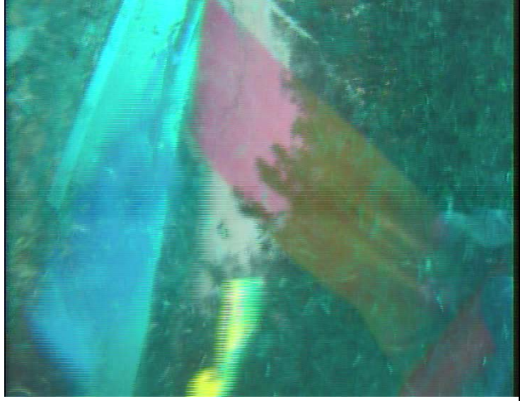
Surface of the pipe after epoxy filler application Feature 1.
