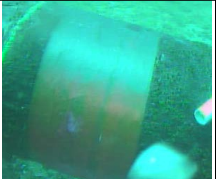
Surface of the pipe after release film application Feature 1.
