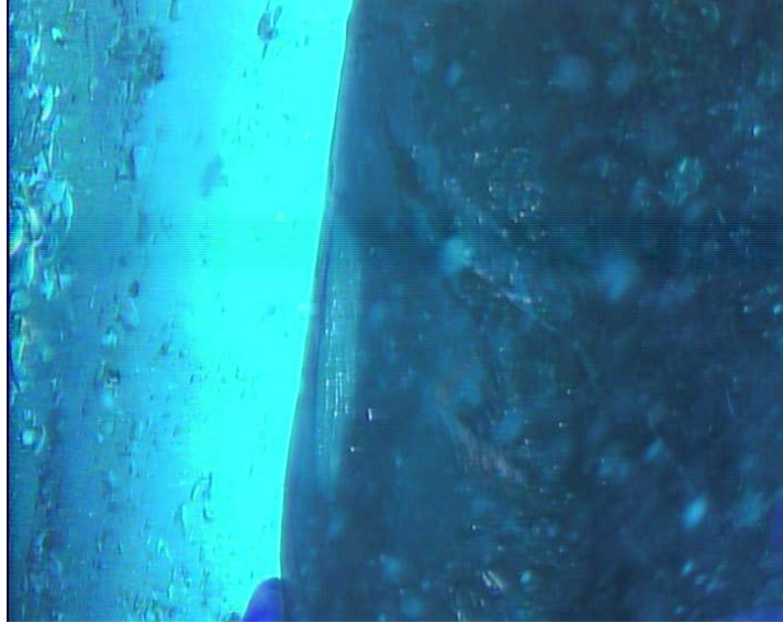
Surface of pipe after surface preparation Feature 1.
