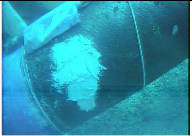
Surface of the pipe after epoxy filler application Repair Area # 8.
