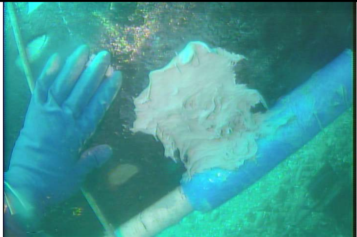
Surface of the pipe after epoxy filler application Repair Area # 13.
