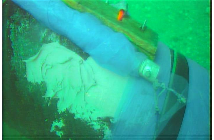
Surface of the pipe after epoxy filler application Repair Area # 7.
