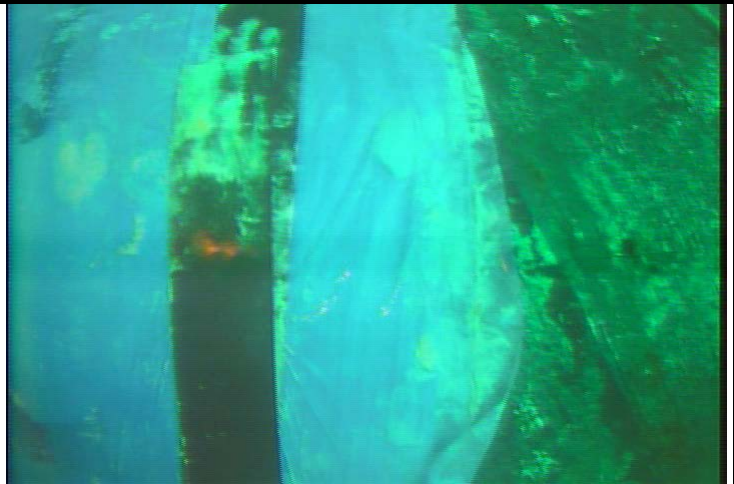
Surface of the pipe after release film application Repair Area # 7.
