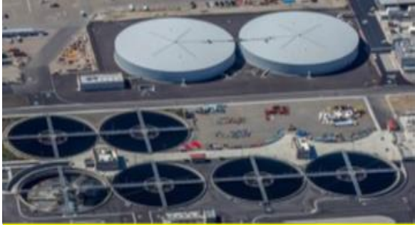
A $135 million WIFIA loan issued to the Orange County Water District will expand the area's drinking water supply. (Orange County Water District photo)
