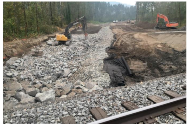
Construction underway to restore stream channel habitat upstream of Puget Sound in Washington. (Image courtesy of NOAA)
