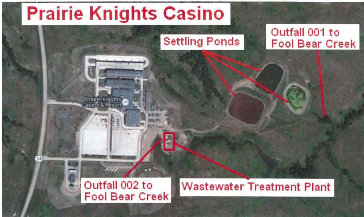
Figure 1- Overview of Prairie Knights Casino WWTP
