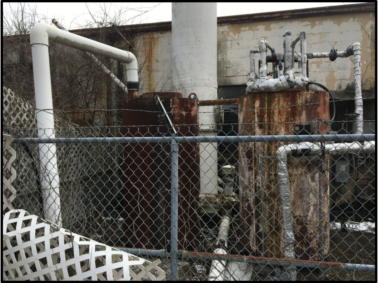
Picture 4: Groundwater Pump and Treatment System
