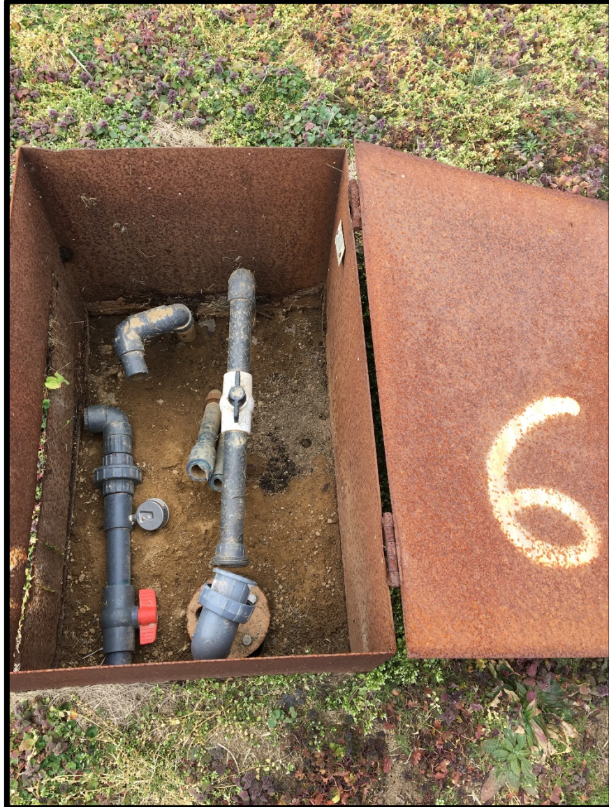
Picture 3: Eductor Well EW6
