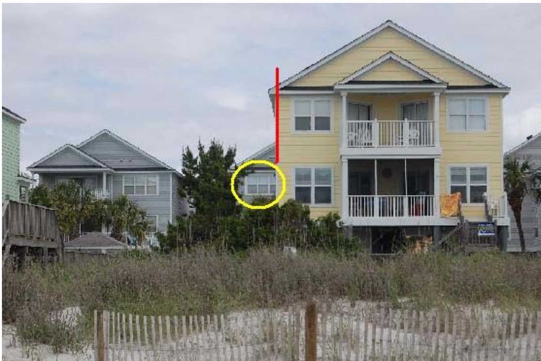
Figure 10a: Right transect (View from the water)
