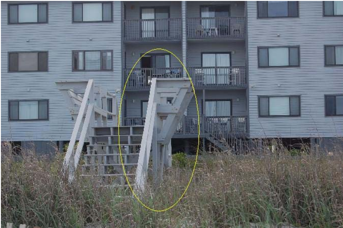
Figure 9c: Center transect (Handrail of Walkway)
