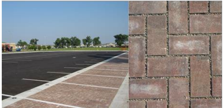
Left: The completed permeable pavement parking lot behind Seitz Elementary School on Fort Riley. Right: When it rains, stormwater infiltrates through the gravel-filled spaces between these pavers into the ground below.
