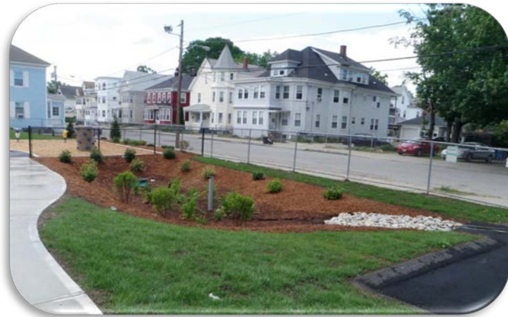
Bioretention system in Lawrence, Massachusetts, installed during the redevelopment of a public school site.
