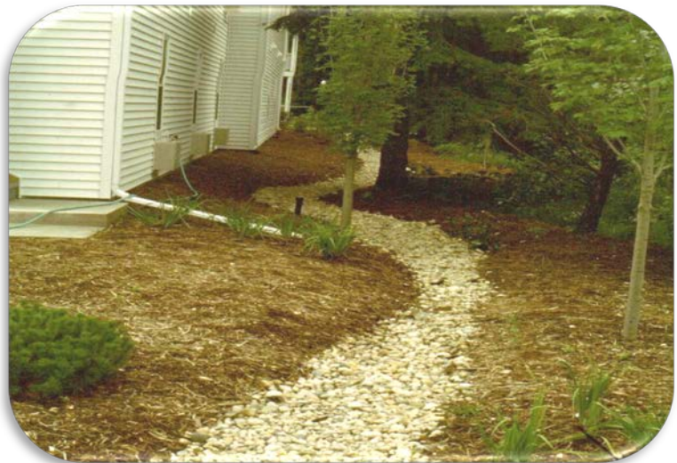
Infiltration trench to recharge roof runoff.
