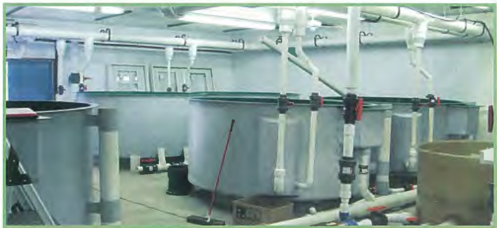
New recirculating tanks at the KBIC fish hatchery
