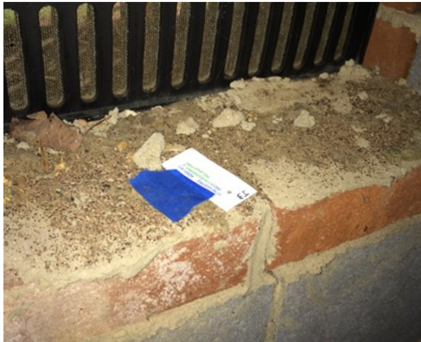
Figure 5-12. BI Disc Package Placement at Periphery of Crawl Space
