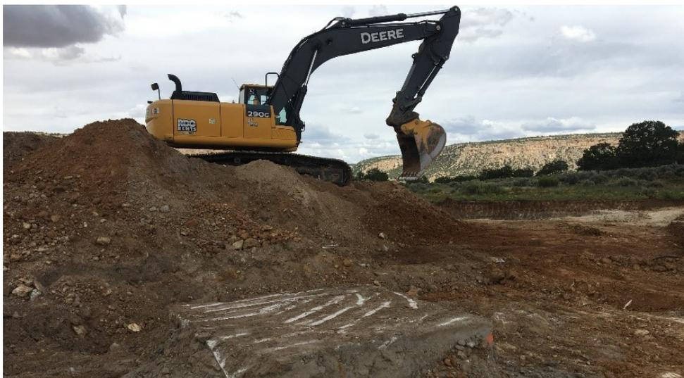
*Excavating contaminated soil near a ventilation shaft during the 2017 Quivira Removal Acton. The cement cap on the ventilation shaft is in the foreground.*
