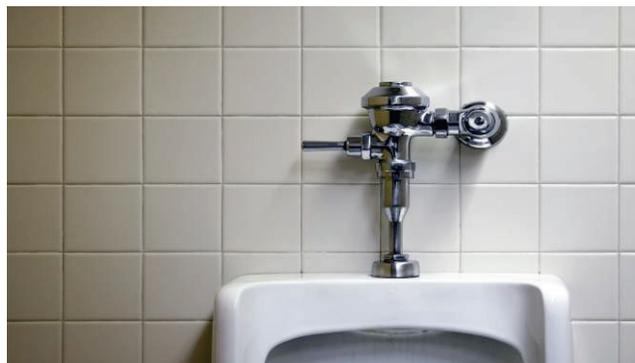
Each WaterSense labeled flushing urinal can save a facility more than 4,600 gallons of water per year.
