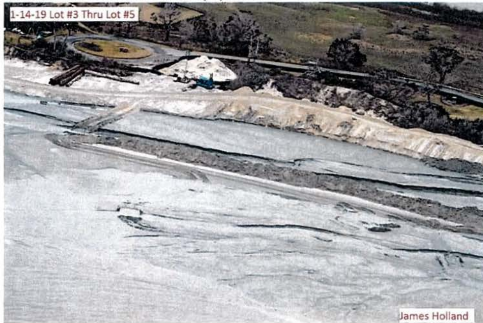
Photo No. 4 – This January 14, 2019, photo shows sand being stored near the road outside of permitted construction area for Lot Nos. 3, 4, and 5.
