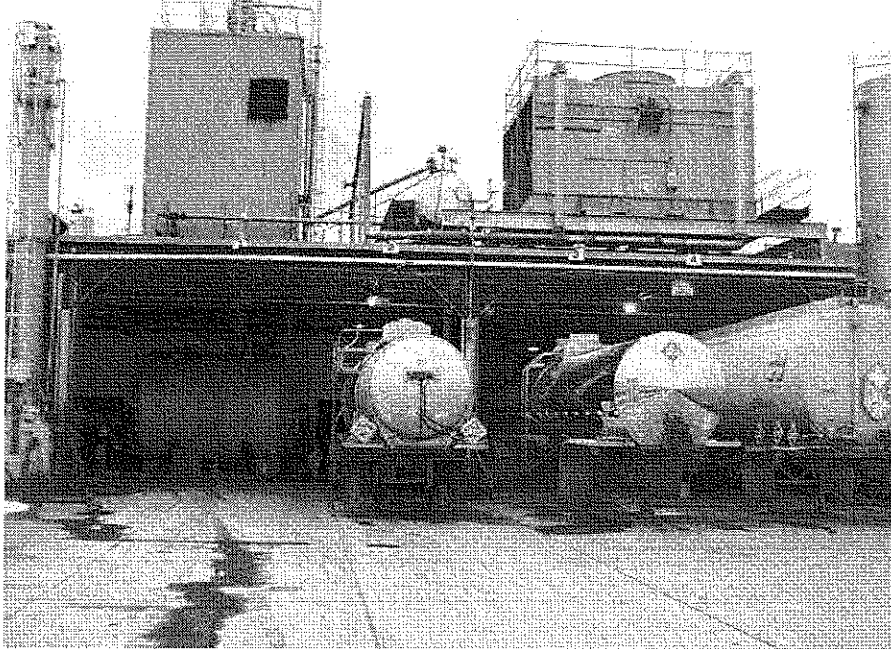
East Pad Area - Bulk Fuels
