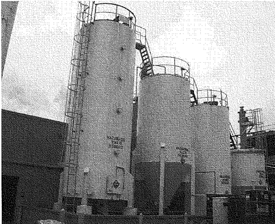
F-1 Tank Dike Area – “Chemfuel” Tanks
