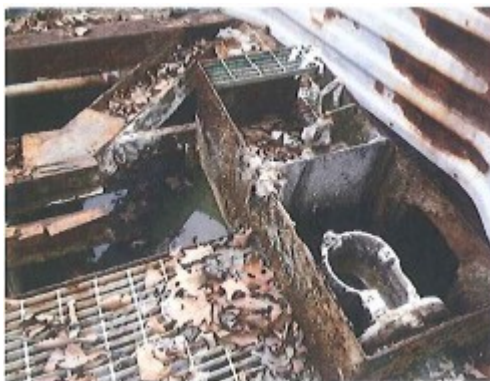
Mountainaire Package Plant, April 2016
