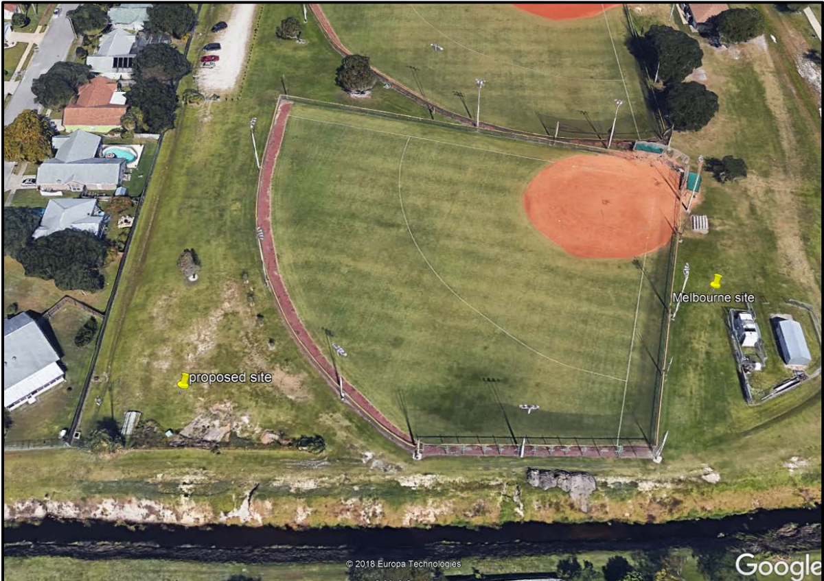
Figure 3.5 Aerial of Original and Proposed Melbourne Site Locations
