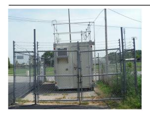
The monitoring site is a stationary equipment shelter located in a fenced-in area near the intersection of Second and Carpenter Streets in Shepherdsville, Kentucky. The sample inlets are 56 meters from the nearest road. Upon inspection, the sample lines and monitors were found to be in good condition. The site meets the requirements of 40 CFR 58, Appendices C, D, E and G.
