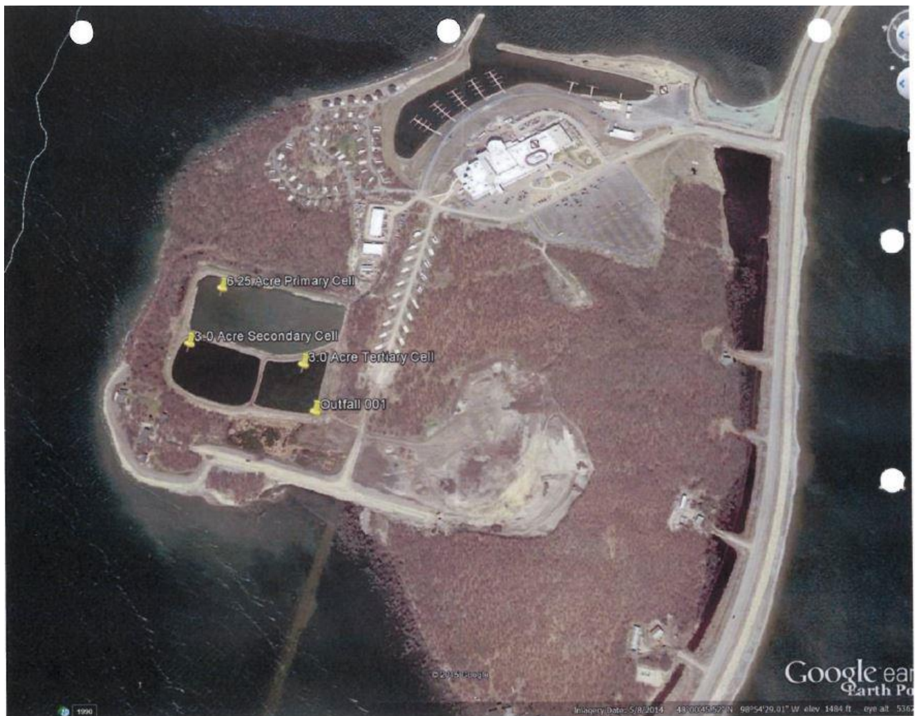
Figure 1. Spirit Lake Casino WWTF
