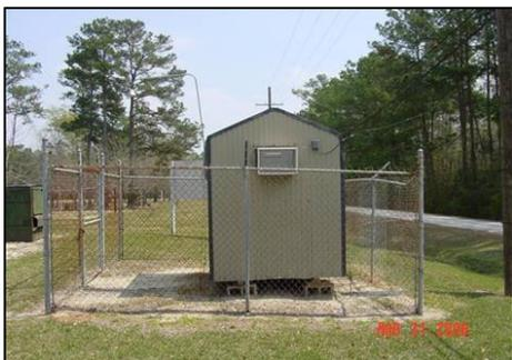
The Bushy Park Pump Station site is located in southeastern Berkeley County downwind from the Charleston urban area. This site monitors for Ozone and the monitoring objective is maximum Ozone concentration. The sample inlets are 15 meters from the nearest road.
