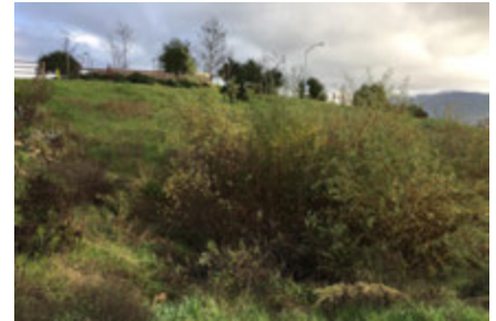
This 300-yard-long bioswale on the Santa Ynez Reservation in California is designed to reduce flooding danger to surrounding homes. It also provides wildlife habitat.
