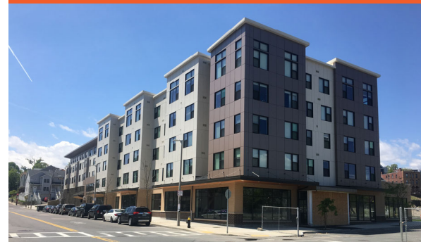
Figure 2: Bartlett Station Apartments Credits: Nuestra CDC
