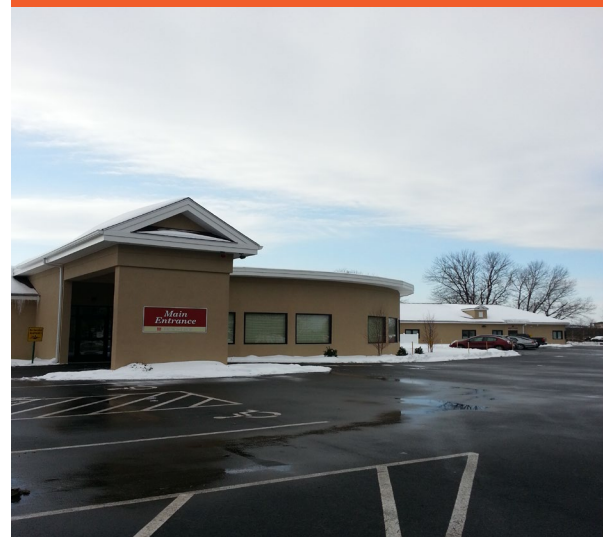
Figure 2: Main Entrance Credits: City of Manchester
