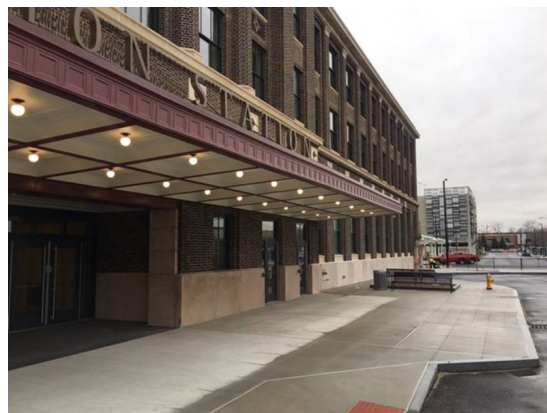
Figure 1: Front Entrance Credits: EPA
