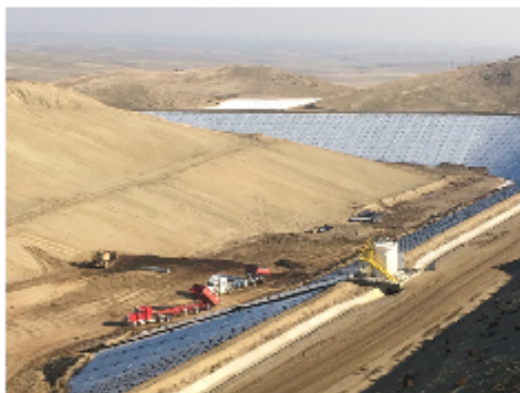
Kettleman Hills hazardous waste landfill.
