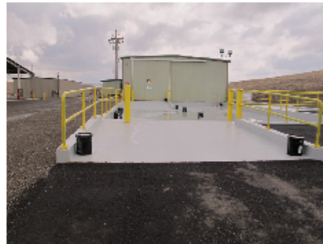
PCB storage building at Kettleman Hills facility.
