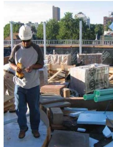
*Image 15.1, Example of temporary dead and live loads during installation at the Gathering Place, Denver.
