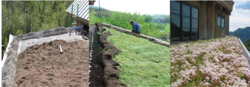
*Photo 27.1 Example of 12" vegetation free zone at the perimeter of a green roof with vegetation mat. Photo on the right is one month after installation.*
