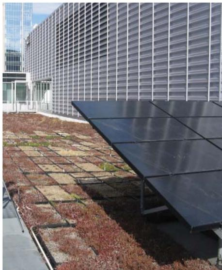
*Image 30.1 Integration of solar panels on a green roof. EPA, Region 8, Denver.*
