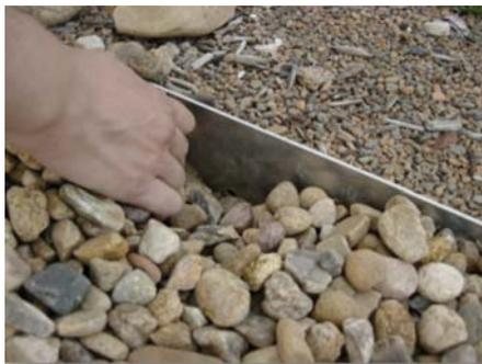
*Image 22.1. Stainless steel plate around the perimeter of a roof drain*
