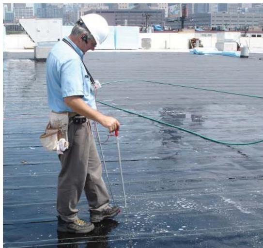
*Photo 29.2 Example of flood electric field vector mapping*
