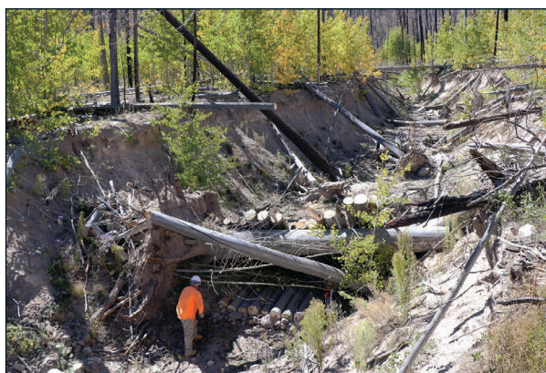
A member of the Pueblo of Santa Clara constructs a log mattress and log dam in one of the flood-eroded drainages in the fire-damaged Santa Clara Creek watershed.
