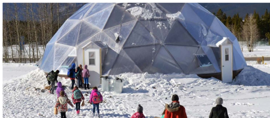
Before and after construction of Growthdome. Cloud City Farm, Leadville, Colo.
