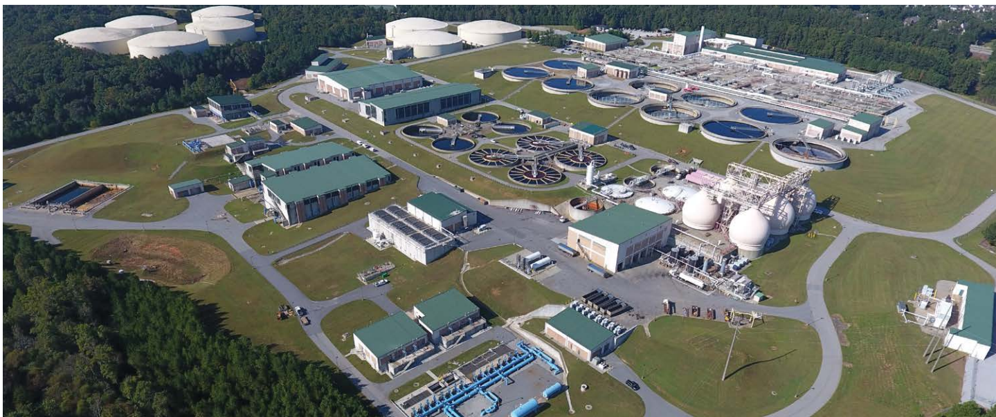
The F. Wayne Hill Water Resources Center in Gwinnett County, Georgia, treats up to 60 MGD of wastewater effluent for surface water recharge to Lake Lanier, while also recovering phosphorus and methane gas.
